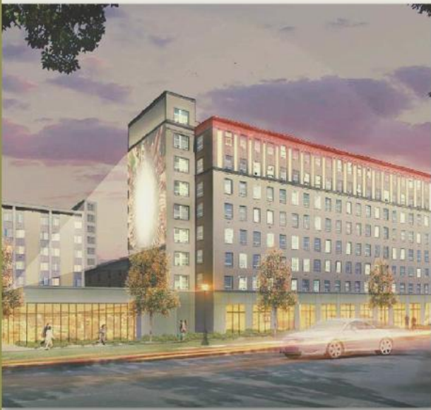
Delmar Divine: A gathering place built for community practitioners and diverse stakeholders.
